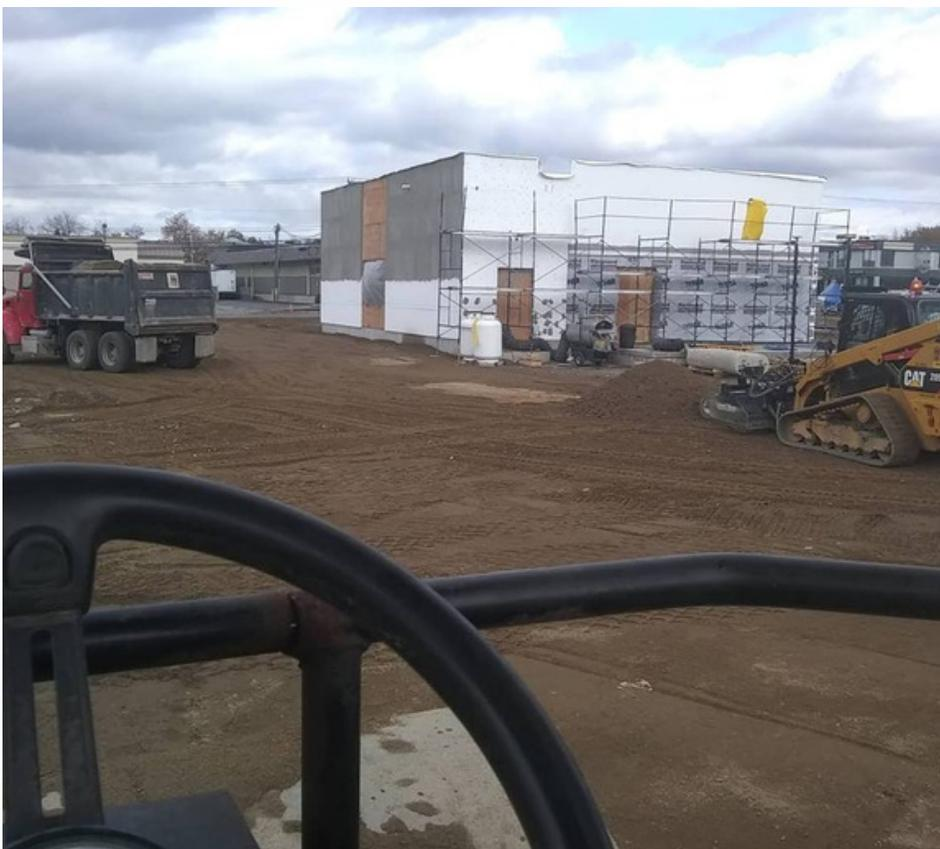
This fall, R.F. Jordan put the finishing touches on the new Dairy Queen building on High Street in Ellsworth, working with the general contractor Nichols Construction to fill, grade, and pave the parking lots, build and grade sidewalks and a patio, install lighting and drive-thru menu sign posts, and site drainage. The restaurant has an anticipated opening in December 2018, and we will return in the spring of 2019 to put the finishing touches to the site.
