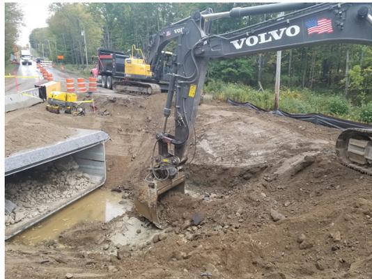
As part of their continuing mission to maintain and upgrade Maine's transportation infrastructure, the Department of Transportation contracted with R.F. Jordan to install a new box culvert on Route 46 in Eddington. The new culvert is 6' tall, 16' wide, and spans the entire width of Route 46, carrying a stream safely underneath the roadway. Plans are in the works to install a similar culvert on Route 46 in Bucksport in 2019.
