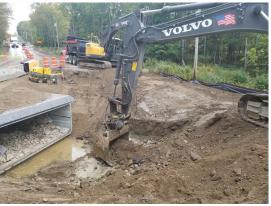
As part of their continuing mission to maintain and upgrade Maine's transportation infrastructure, the Department of Transportation contracted with R.F. Jordan to install a new box culvert on Route 46 in Eddington. The new culvert is 6' tall, 16' wide, and spans the entire width of Route 46, carrying a stream safely underneath the roadway. Plans are in the works to install a similar culvert on Route 46 in Bucksport in 2019.
